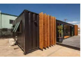
The container itself was fitted with fins on the outside panels and welded to the facias so not to impeach the integrity of the container walls which could lead to the ingress of water. It was then clad in fireproof coated timber as well as the doors and the louvers disguised behind timber grills to remain sympathetic to the environment and to make the new plant room appear as a timber cabin.
