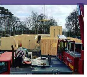
The frame production was then fabricated off-site and Installed on-site. Therefore, the need for cutting or changes were kept to a minimum once on-site.
